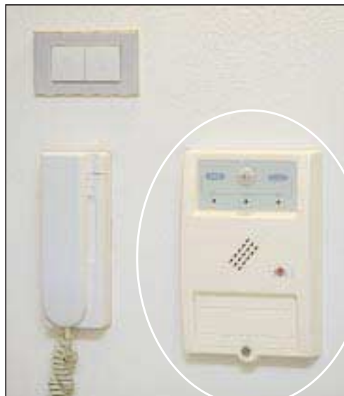
C12 ALARM CONTROL UNIT
